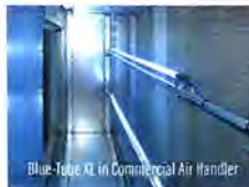
Blue-Tube XL in Commercial Air Handler 2
